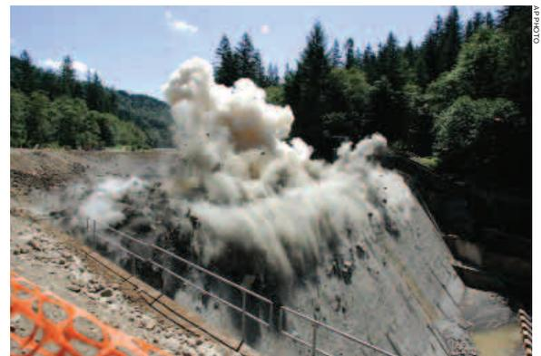
*Explosives blast the first cracks in Marmot Dam July 24.*
